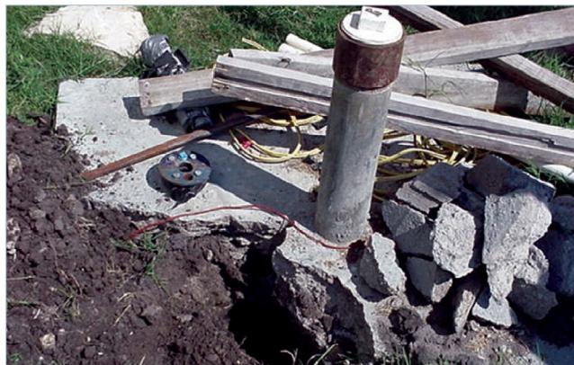
Figure 59. The slab around this well is not sufficient to prevent surface contaminants from entering the aquifer. (Source: *Plugging Abandoned Water Wells*, Bruce Lesikar and Justin Mechell, 2010.)
